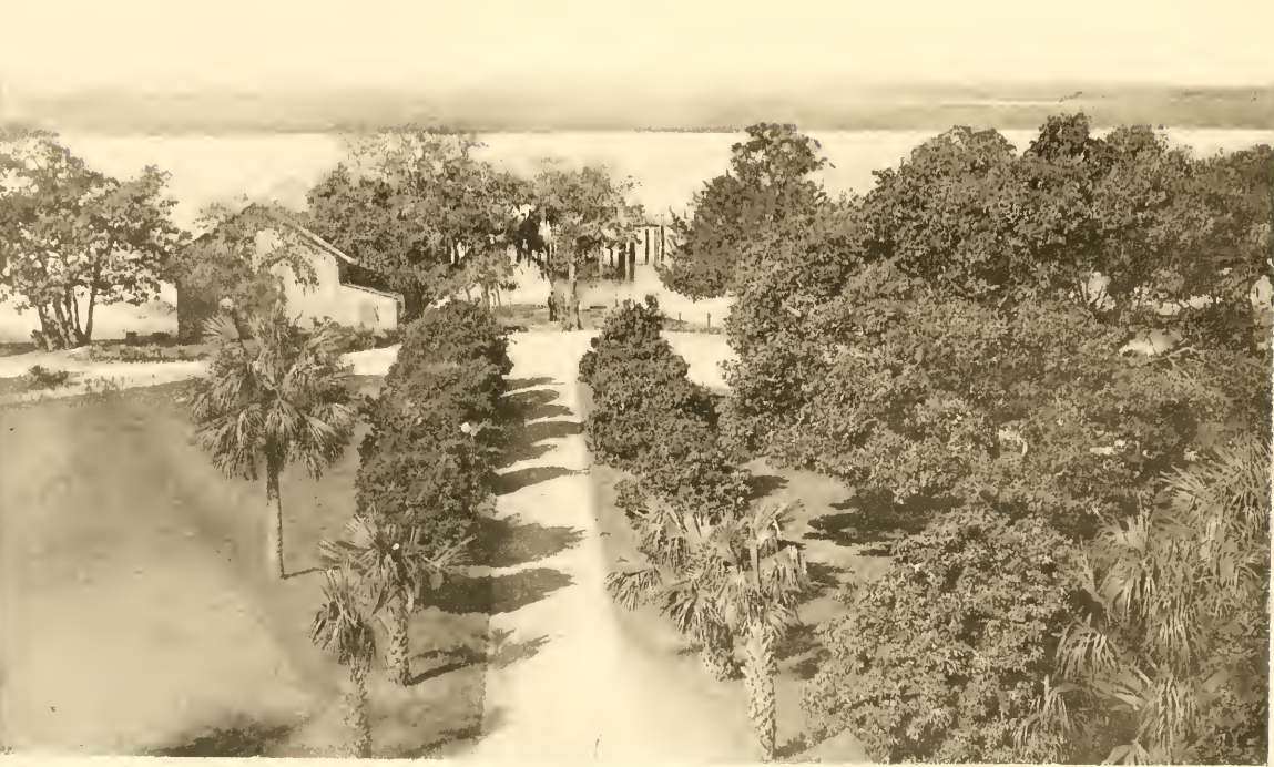
ROAD TO BOAT LANDING
